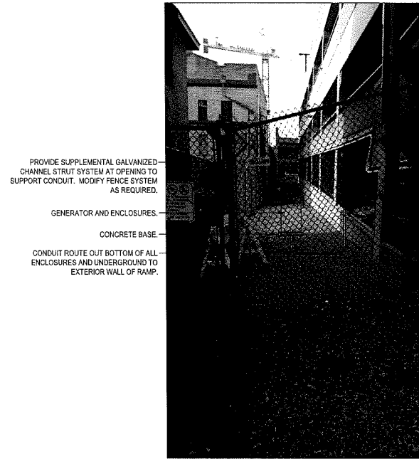
6 GENERATOR RACEWAY DETAIL NO SCALE
